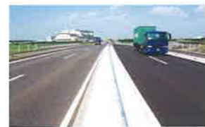
臨港道路鍋田ふ頭進入道路 Seaside Road Leading into Nabeta Pier
