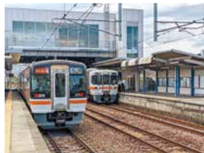
▶ JR 蟹江駅橋上駅舎
