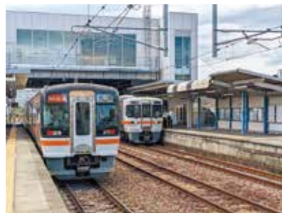
▶ JR 蟹江駅橋上駅舎
